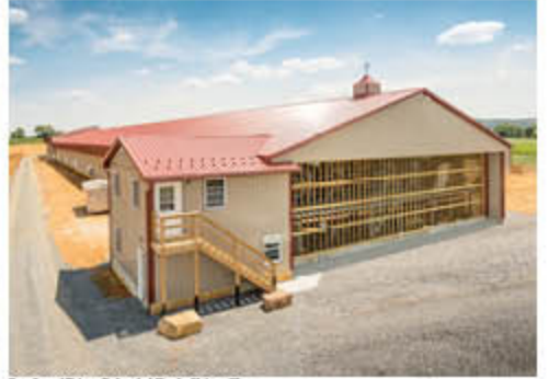
Roof and Trim: Colonial Red Sides: Clay
