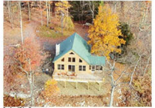
Roof and Trim: Evergreen
